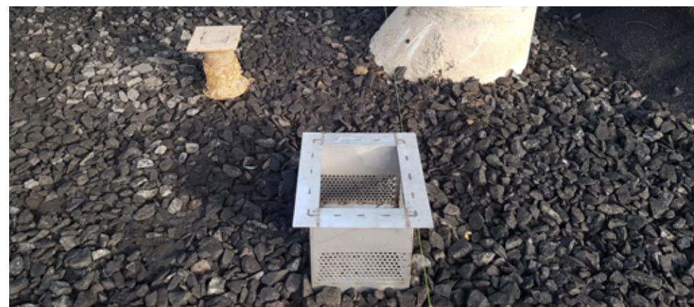
Figure 3: Most of a structural soil is made up of clean stone. After the stone has been compacted, and a soil mix added, there remains a network of interconnected voids between the stones. These void spaces provide opportunities for root growth, air diffusion, and water movement.
